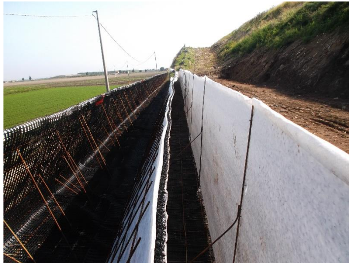
Figure 2: External capping over the retaining structure for waste
