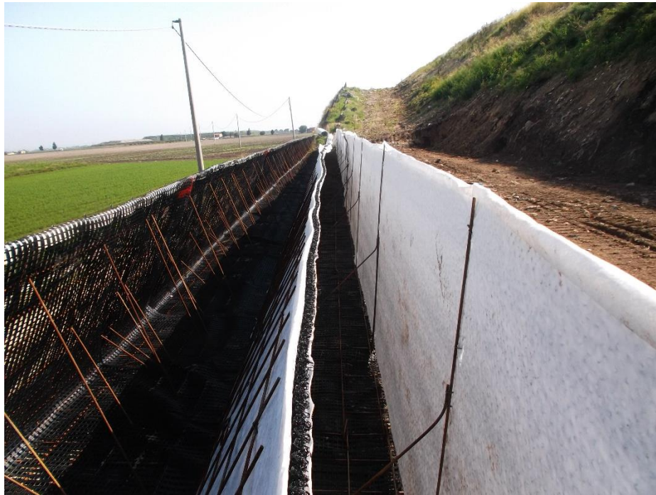
Figure 9: External capping over the retaining structure for waste
